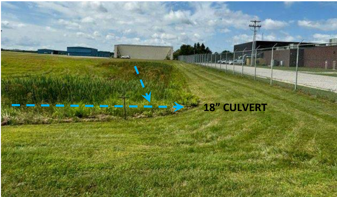
Photograph 3: Southward view where the drainage ditch flows into an 18" culvert under Flight Line Drive. Surrounding slopes have been graded toward the culvert to also capture drainage from the south.
